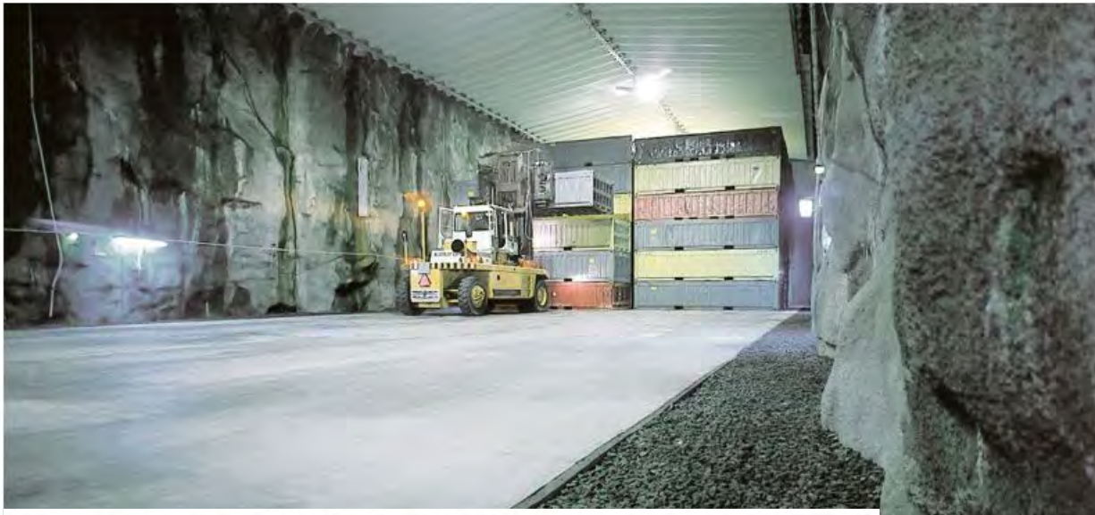
One of the rock caverns for LLW inside Sweden's SFR facility
